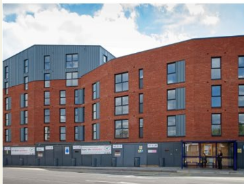
GOLDSMITH AVENUE, PORTSMOUTH
