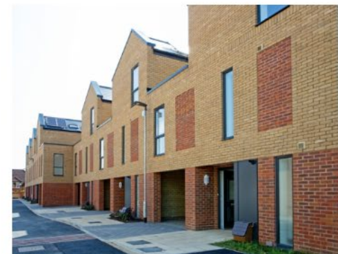
LARGES LANE, EDENFIELD, BRACKNELL
