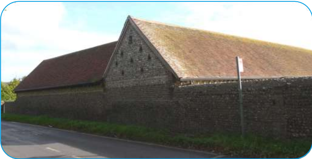
An impressive farm complex sits on the opposite side of the road to Upton Farmhouse and presumably was part of the whole farmstead.
