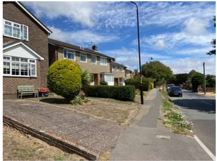
Fig 28: Modern housing on north side of Manor Road west of the church
