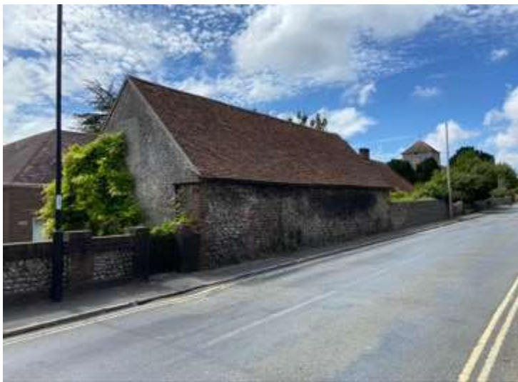
Fig 36: View looking west along Manor Road towards barn and church tower
