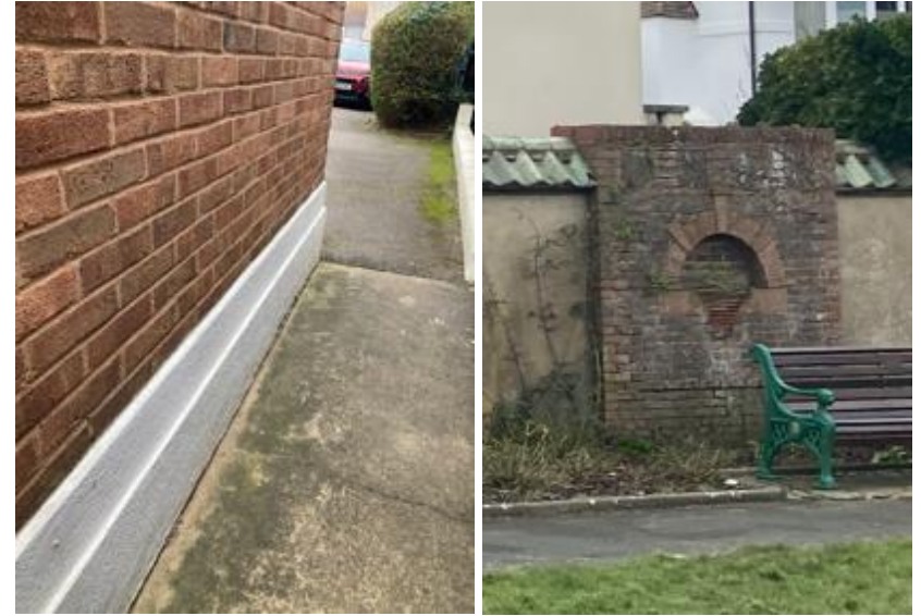
Figure 31: Brickwork at Hastings Court and within locally listed walls of Marine Gardens
