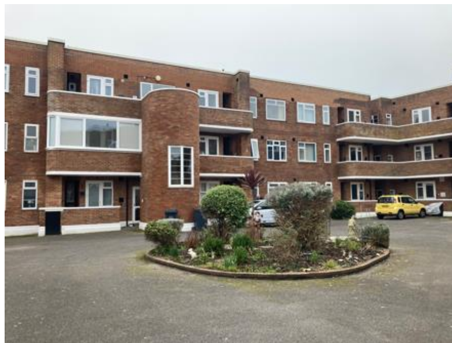
Figure 27: Winchelsea Court, rear elevation
