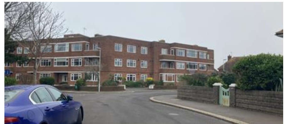
Figure 35: Low brick boundary walls around Winchelsea Gardens
