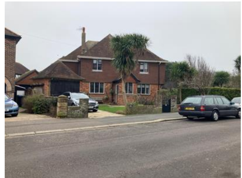
Figure 29: No.2 Dover Road
