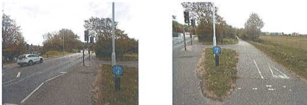
Figure 3 View of Shared Footway / Cycleway along the A259 Goring Street
