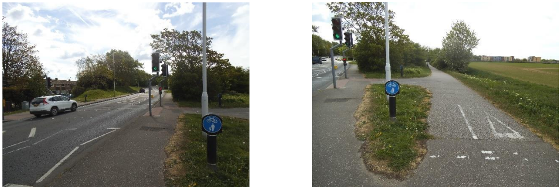
Figure 3 View of Shared Footway / Cycleway along the A259 Goring Street
