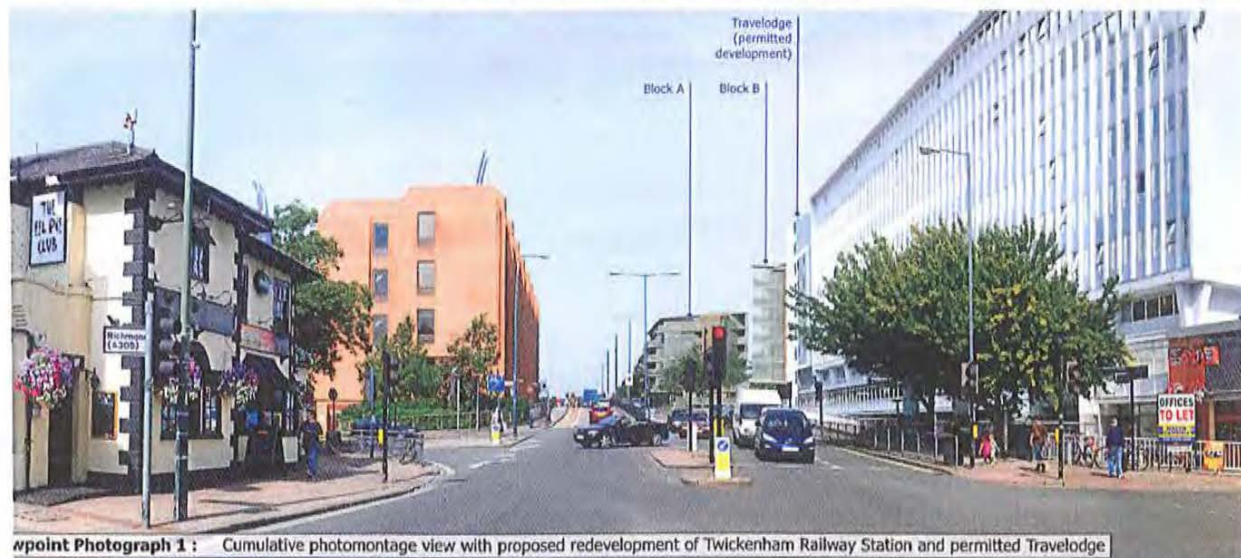
Photograph 1: Cumulative photomontage view with proposed redevelopment of Twickenham Railway Station and permitted Travelodge
