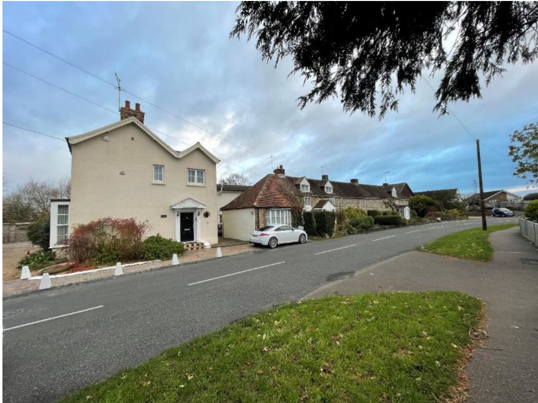
Plate 15: Looking south-east to Clematis and Jasmine Cottages.
