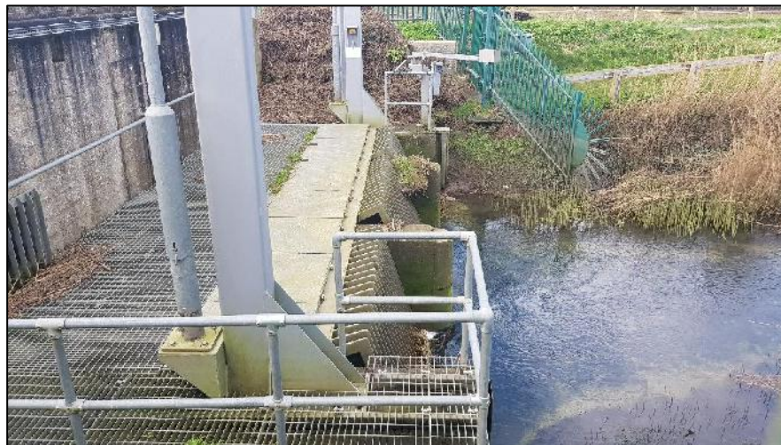
Figure 3: Upstream Face of GOR_1
