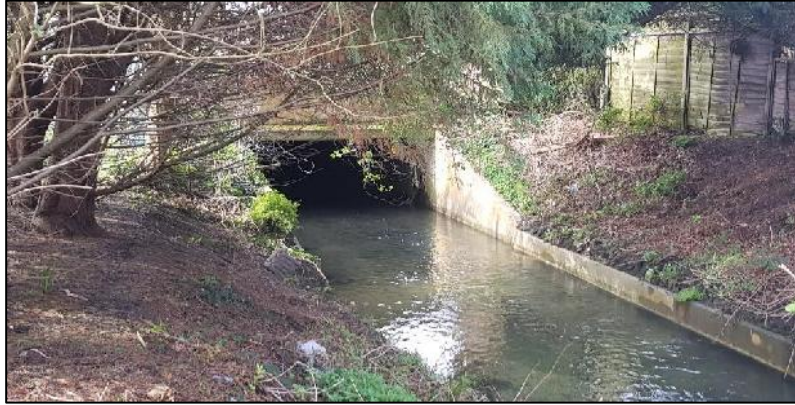
Figure 5: Upstream Face of GOR_2
