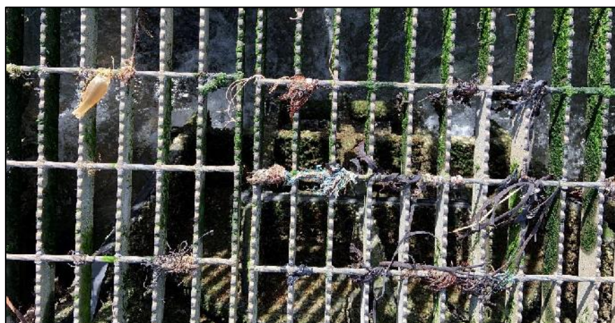
Figure 4: Downstream Face of GOR_1
