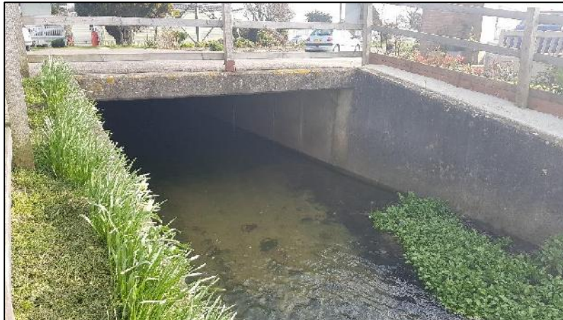
Figure 6: Downstream Face of GOR_2
