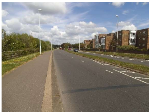
Figure 7 View of A259 Goring Street Adjacent to Site
