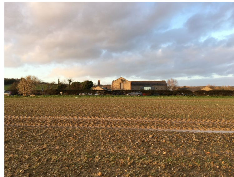
Plate 17 Looking north to North Barn buildings
